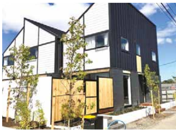
Ozanam Apartments – safe, warm accommodation for vulnerable families.
