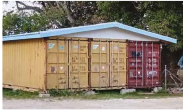
Weatherproof storage containers installed to protect vital supplies.
